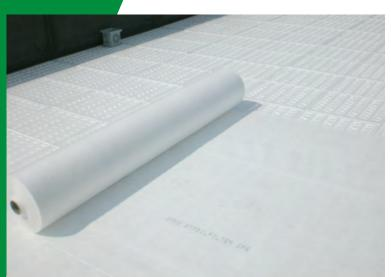
or with contact adhesive, silicone or simple temporary stabilizing mass. In order to protect the stratigraphic to vertical on the perimeters of the waterproofing we recommend lying DAKU STABILFILTER folding it back to the upper limit of the altitude at which the substrate is placed.
